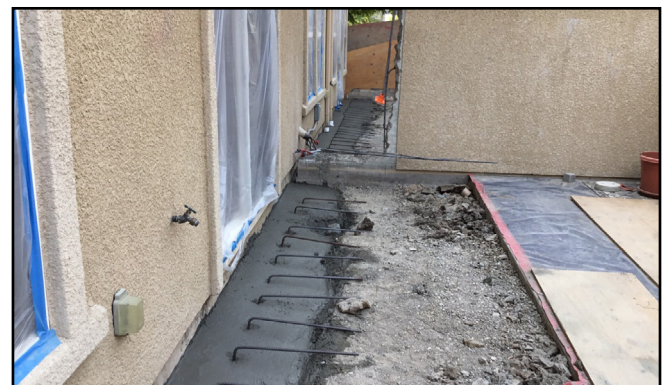
New Concrete Grade Beam, Building 41
