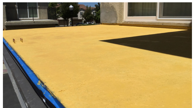
Fiberglass Layer of New Deck Coating System - Building 10
