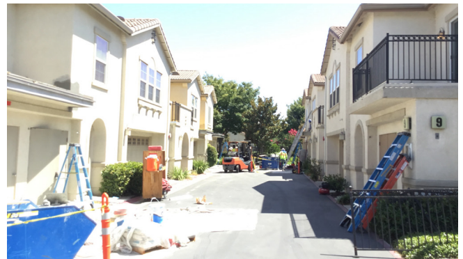
Balcony Repair Work at Buildings 9 & 8
